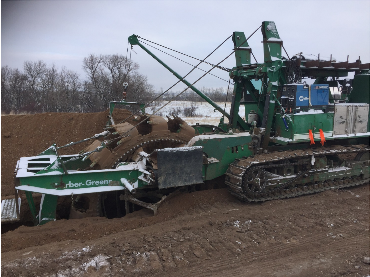
DITCH DIGGING IN THE CLUB ROOT AREA (490)
